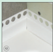
12 Ensure Sealux-N fuses across joints inside strips
