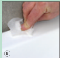
6 Wipe ledge with alcohol or methylated spirits
