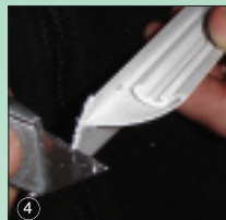
4 Pare off freys at cut ends
