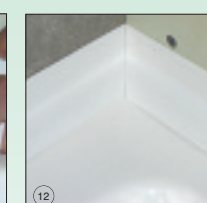
12 Ensure Sealux-N fuses across joints inside strips
