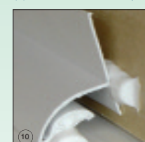
10 Lay Sealux-N on wall as shown. Rotate strip into position over ledge
